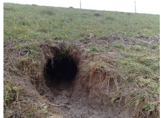
Figure 13, hole in a dike burrowed by a beaver
